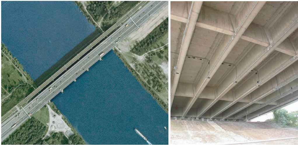
Figure 1: (left) Aerial picture of the situation of the Hollandse Brug, which connects the ‘island’ Flevoland to the province Noord-Holland, and the adjacent railway bridge. (right) Some of the sensors attached to the underside of the bridge.
